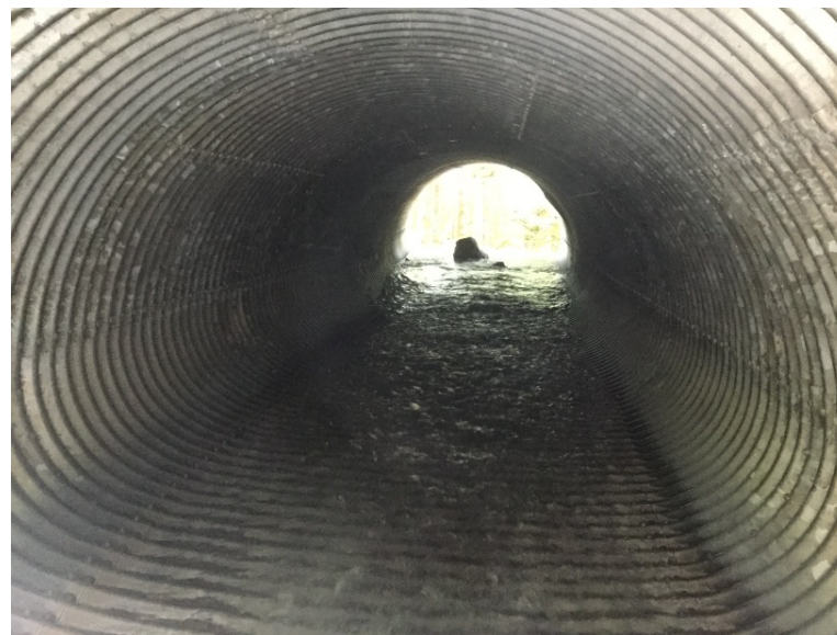
Looking through culvert from inlet
